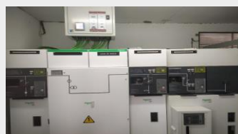
Grid connection 20 kV
