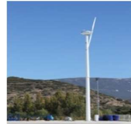
Wind turbine, 20 kW
