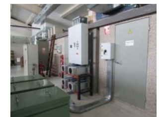
Supercapacitors, 30 kW, 45 s
