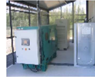
Diesel generator, 55 kVA
