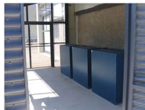
Programmable loads 120 kVA
