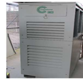
Gas microturbine, 30 kW
