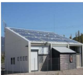
PV system, 25 kWp
