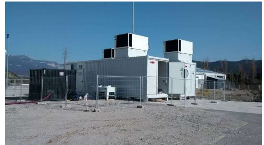
Ion Lithium Battery 1 MW, 500 kWh.
