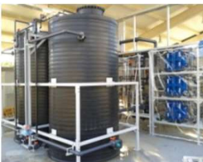
Flow battery, 50 kW, 4 hours
