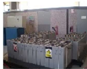
VRLA batteries, 50 kW, 2 hours
