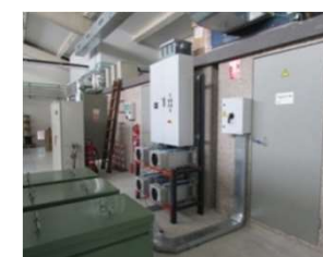
Supercapacitors, 30 kW, 45 s
