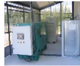
Diesel generator, 55 kVA
