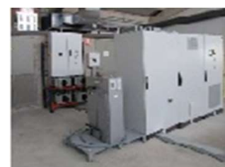
Li-ion battery, 50 kW, ½ hour
