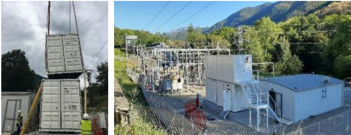
Installation of the storage & control system at RTE substation
